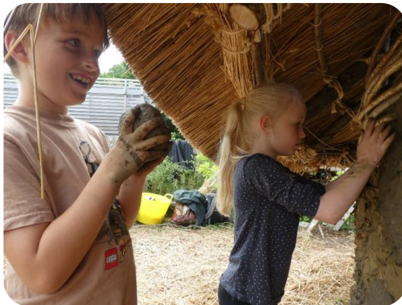
Bronze Age Roundhouse construction & related workshops
